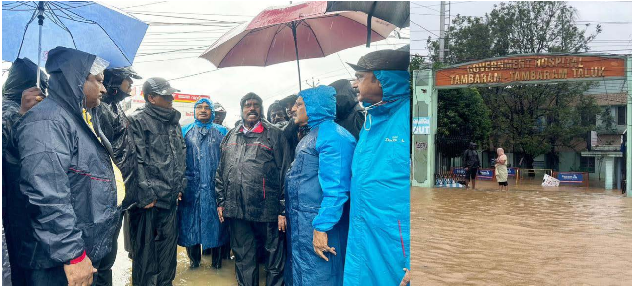
Hon'ble Minister for Public Works, Highways and Minor Ports inspected the flood affected GST road at Chromepet near Government General Hospital- Chengalpattu District
